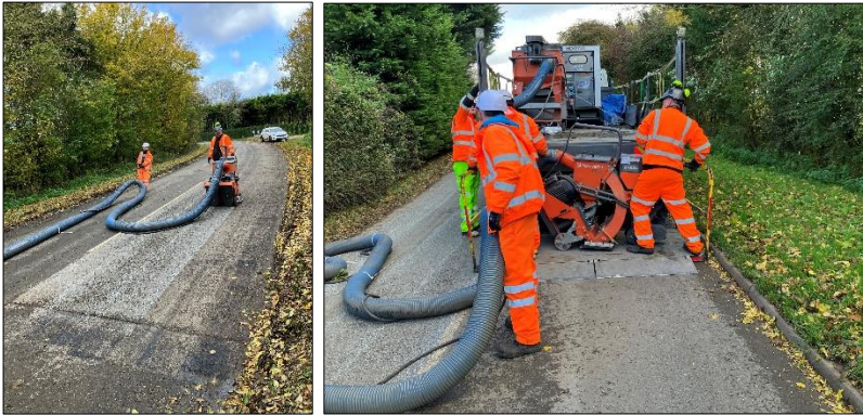
Road retexturing can be a quick, effective and low-cost method of restoring skid resistance to roads.
